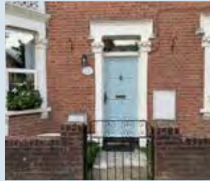
Wooden door and frame details
