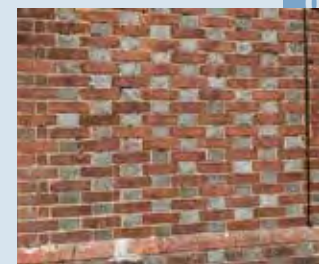
Brickwork in Flemish Bond
