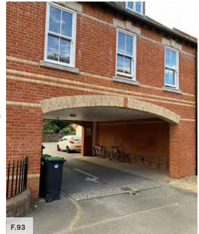
Figure 93: Courtyard parking on Fairfield Road. The courtyard parking can be softened by proposing adequate landscaping
