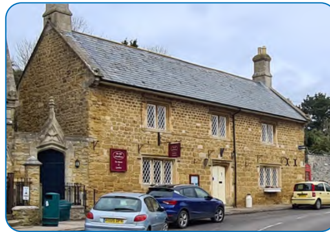
Figure 40: Grade-II listed - Detached Schoolmaster's House, rubble-stone walls, squared and coursed. Slate roof with stone gable-copings and moulded stone kneelers. Stone stacks at each gable.
