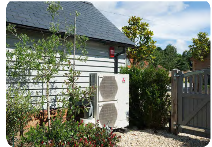
Figure 64: An example of air source heat pump
