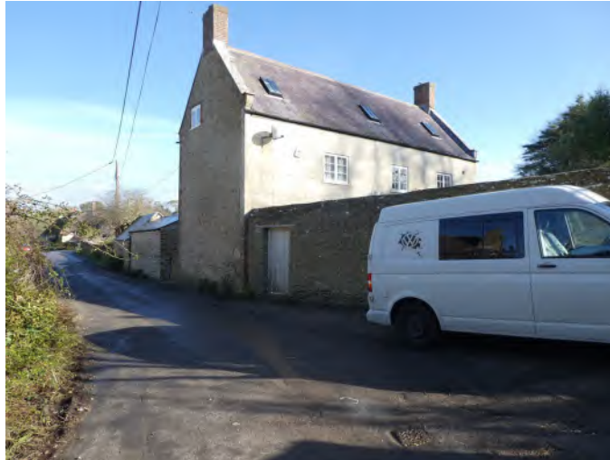
Figure 8: Higher Farm Cottage with siltstone and plain tile and double Roman pantile
