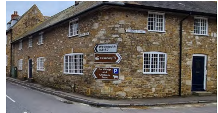
Figure 21: A rubble-stone corner cottage with rounded corner.
