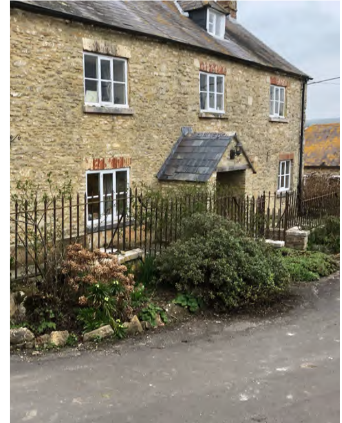
Figure 10: Lower Farmhouse with rubble stone walls with slate roof with gable ends
