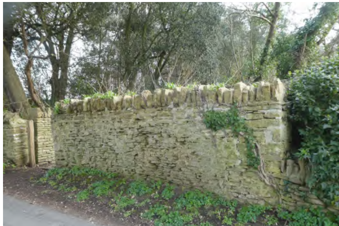
Figure 9: Village pond with stone wall made by shallow rubble-stone and vertical coping stones
