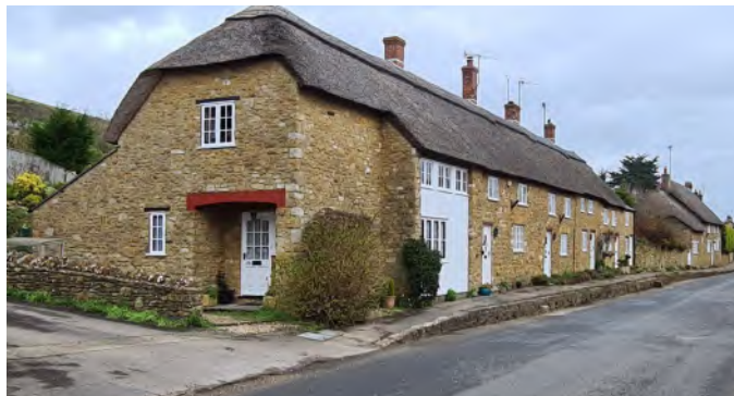
Figure 19: Four cottages in a row with rubble-stone walls, white render and thatched roof with wooden casement window
