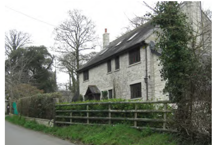
Figure 6: Two-storey house with stone and slate roof with sunlight and gabled porch
