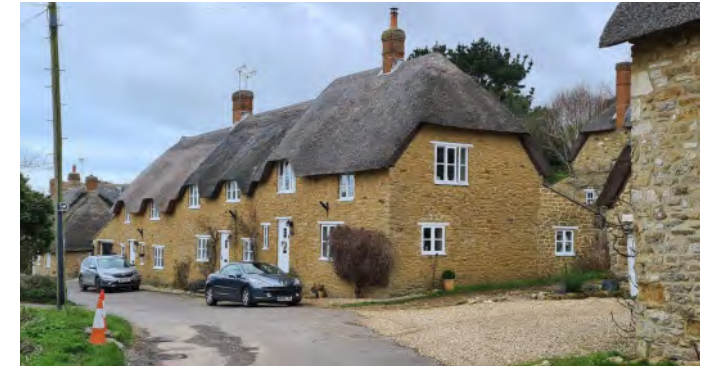
Figure 20: A row of thatched roof cottages with stone walls
