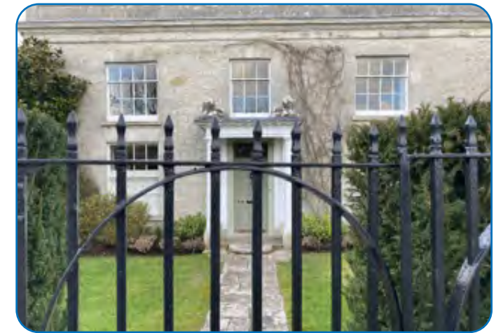
Figure 39: Grade-II listed Portesham House - A detached house with coursed rubble-stone walls and dressed stone quoins. Stone slate roofs with gable-copings
