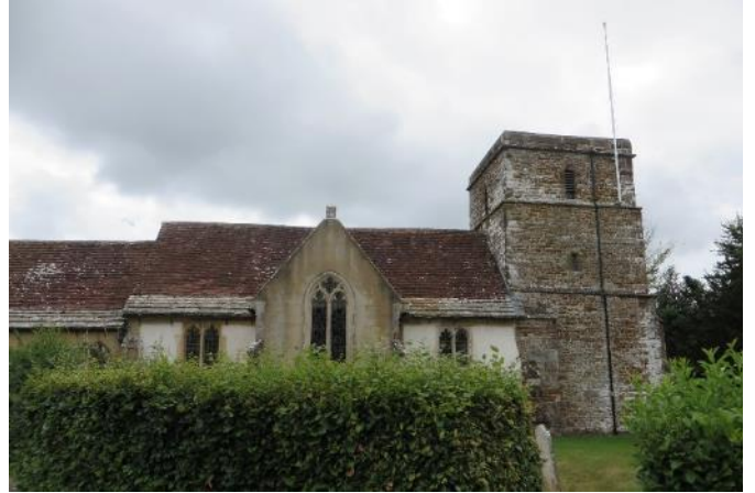
The grade II* listed Church of St Hubbard, situated to the north-west of the main settlement at the junction of Blandford Road and the A31.
