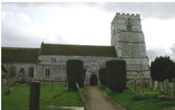
Figure 6: View of Cranborne Parish Church from the north .
