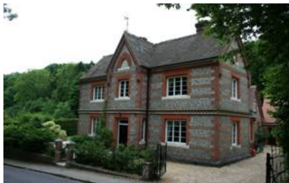
Figure 17: Former Cottage Hospital.
