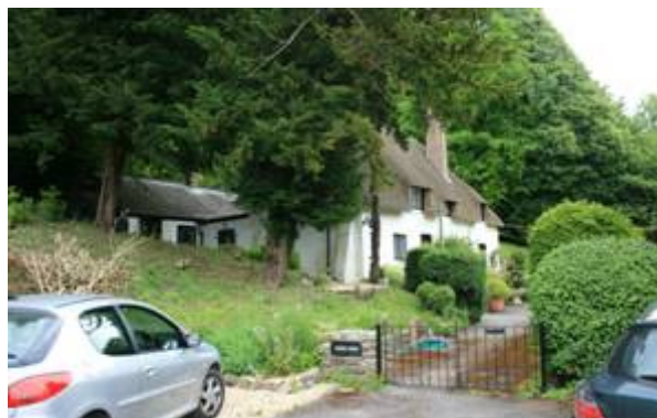
Figure 11: Green Walk, the only surviving house from the old town of Middleton.
