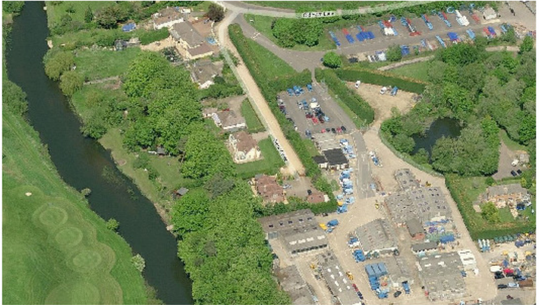
3. Aerial View looking North at existing Depot and Stour Close
