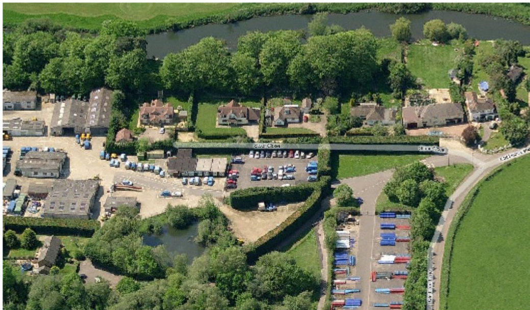
2. Aerial View looking West towards existing Depot and Stour Close
