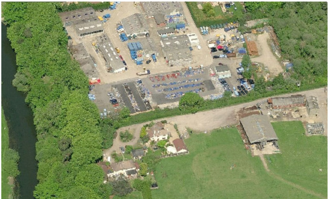
4. Aerial View looking North towards existing Depot
