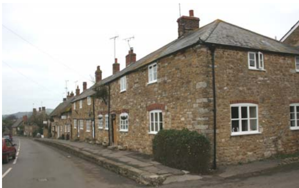
Figure 55: View west along Rodden Row.
