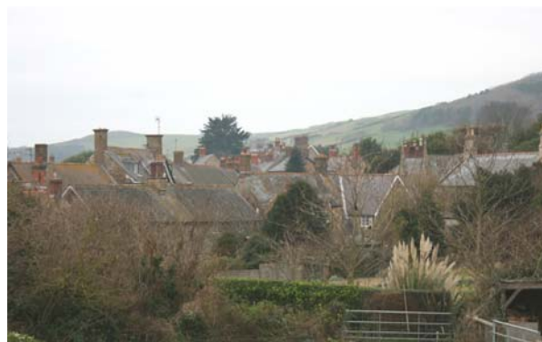
Figure 58: Market Street roofscape.
