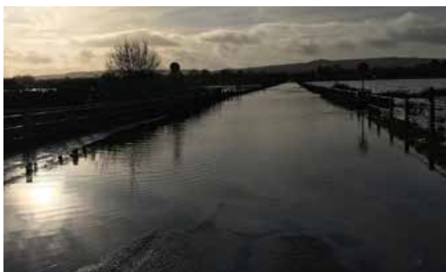
Figure 12: South Causeway Road Flooded January 2020
