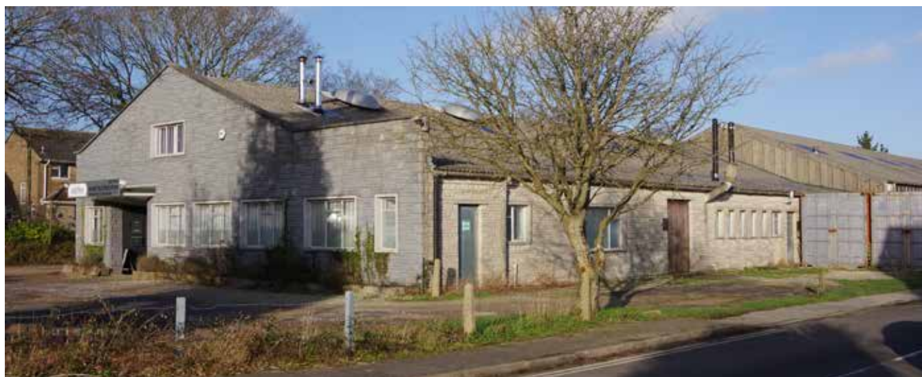
Figure 23: Johns Road Industrial Estate
