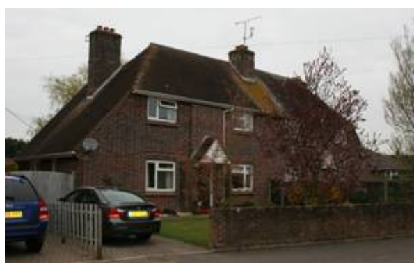
Figure 44: Inter-war suburban housing, 13 and 14 Friars Moor .
