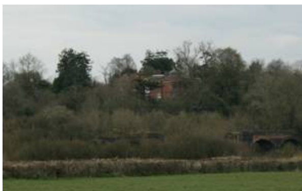
Figure 35: View of Bonslea House with former railway bridge in the foreground.
