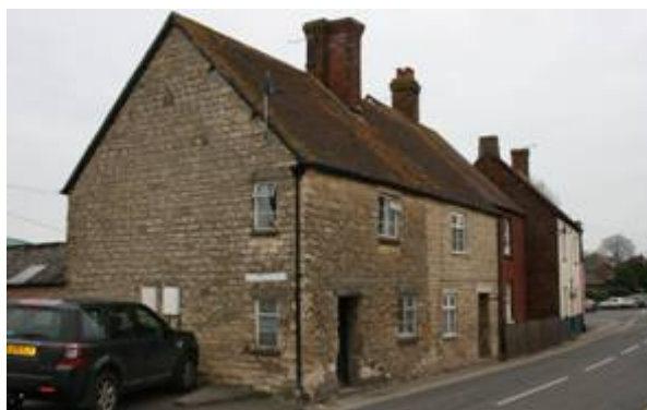
Figure 36: View of Pond Cottages, Butts Pond.
