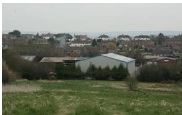
Figure 45: View of Butts Pond Industrial Estate looking south with Rixon Hill in the background.
