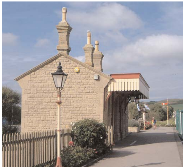
The old station building could be a small refreshment / information shop.
