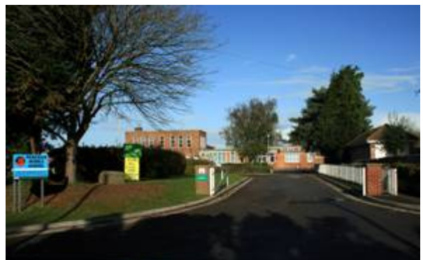
Figure 118: Wareham Middle School
