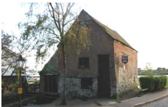
Figure 16: Place Mill, medieval masonry can be found in the stone plinth.
