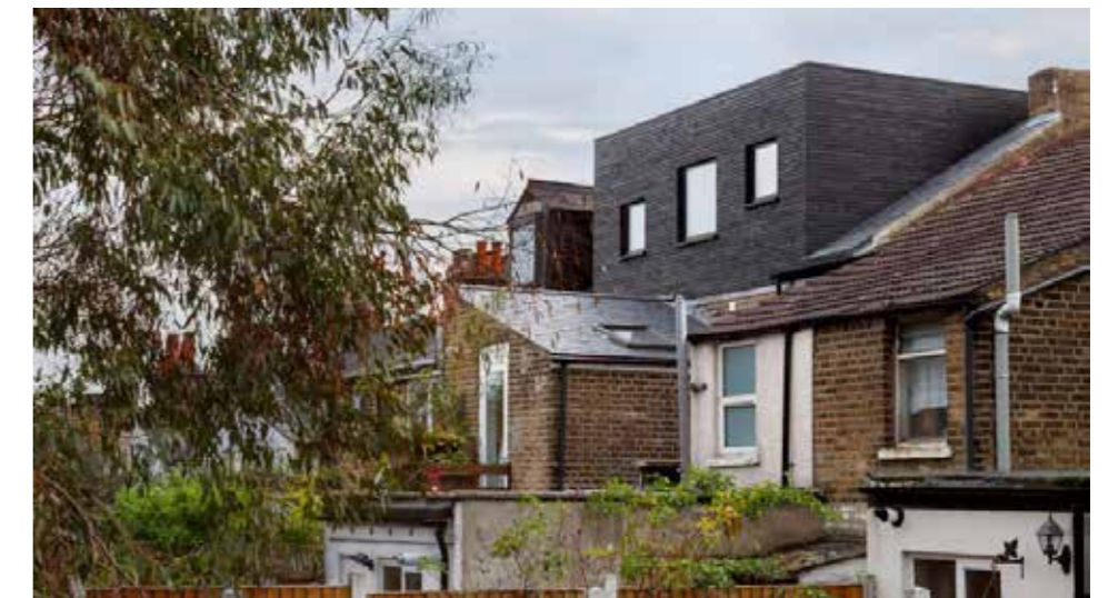
Example showing a jarring extension that goes against existing roof forms and proportion.
