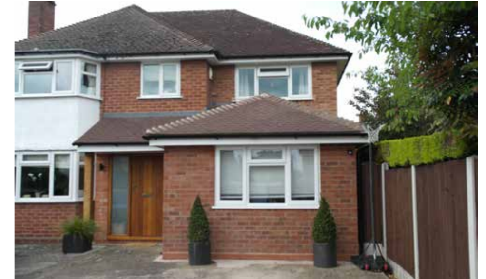
Example showing a front extension with reference to the existing roof and proportion of windows.
