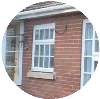
MASONRY DETAILING/ STONE SILL
