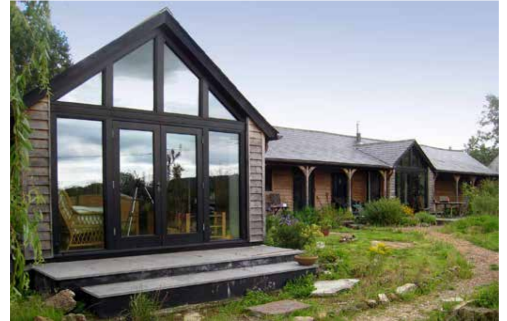
Old Granary, Motcombe. Conversion of cow shed to family home. Western Design Architects
