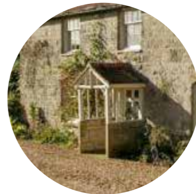
WOODEN/ BRICK PORCH
