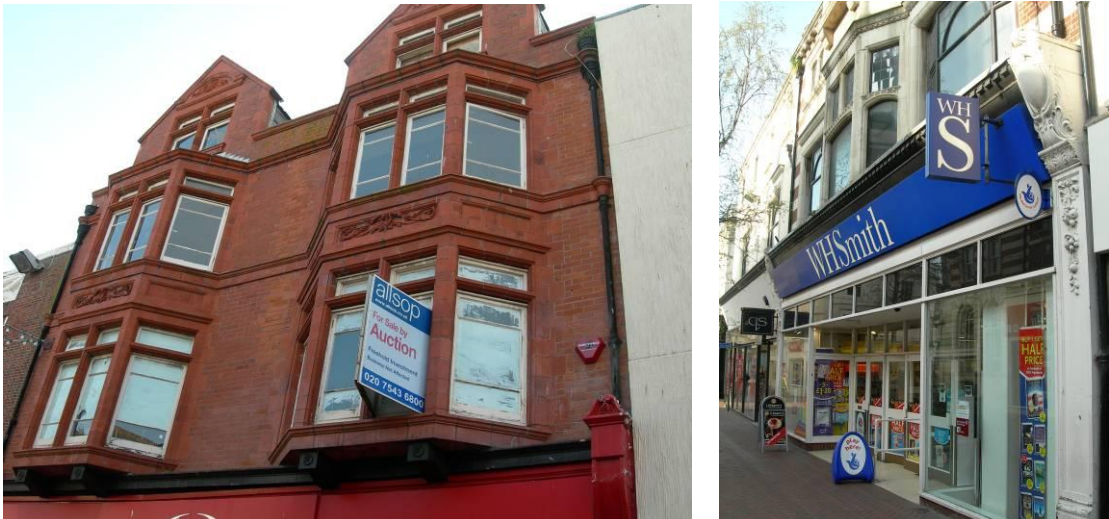
↑ ↗ Examples of underused upper floors in Town Centre buildings
