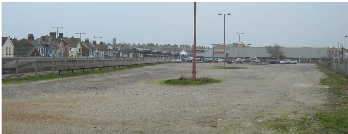
↑ Coach park at Jubilee Sidings – a development option to expand the Town Centre northwards
