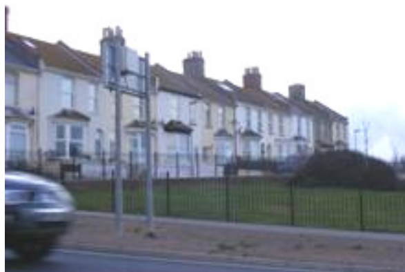
Figure 64: 'Ferrybridge Cottages', workers housing built for the Whitehead torpedo Works
