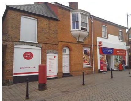
Example of poor colour scheme, inappropriate signage, materials and design. Inappropriate painting of brickwork
