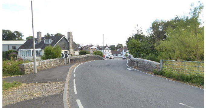
Parapets and rubble wall of listed bridge NHLE ref: 1324445 looking southwest
