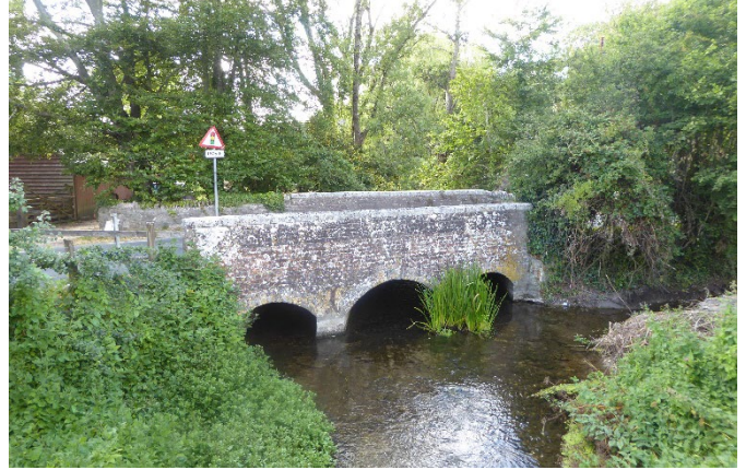
Figure 4.9: The northerly listed bridge (NHLE ref: 1324446) looking northwest
