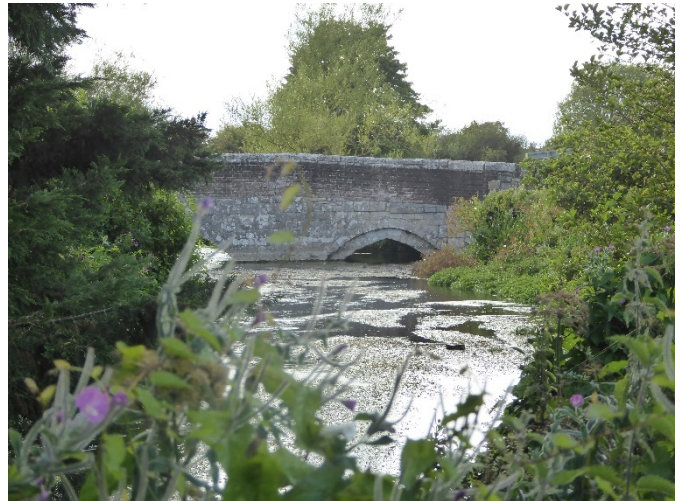
Figure 4.20: Eastern face of Bridge over River Frome on A37
