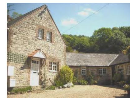
Fig 18 The Old Laundry (left) & Garden Cottage (right)
