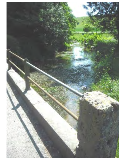
Fig 27 Railings of road bridge near Steepleton Manor entrance
