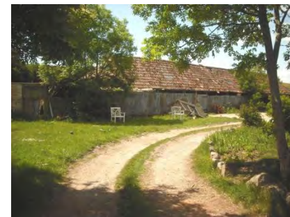
Fig 21 Long shed at Steepleton Farm
