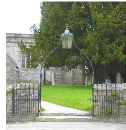
Fig 24. Churchyard gates and lamp overthrow
