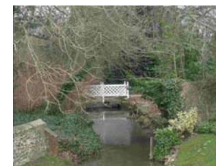
Fig 23. View of River Piddle & footbridge from Rectory Road
