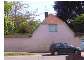
Fig 20. Hayloft & tiled capped cob walls of No 5 Rectory Road
