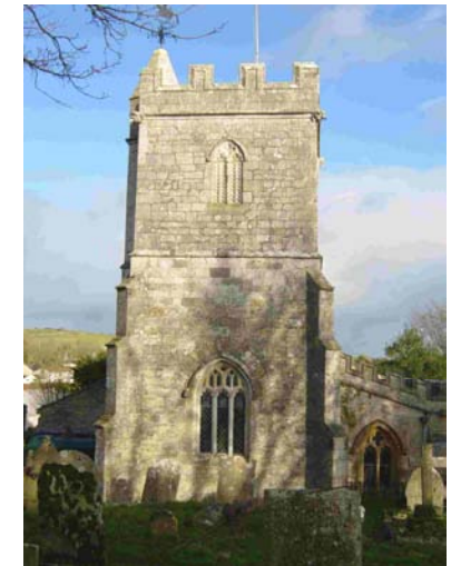
Fig 13. Church tower constructed of Ridgeway stone that is used throughout the village.
