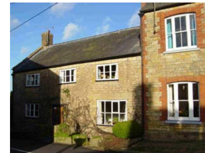
Fig 35. Windows at Belmont & No 1 Fore Place
