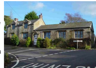
Fig 28. The Old School House
