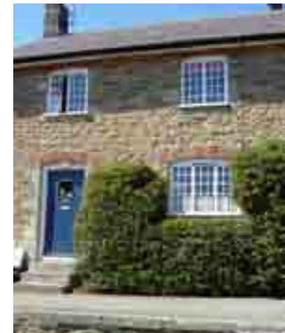
Fig 67. No 36 West St with multiple glass panes and boarded door
