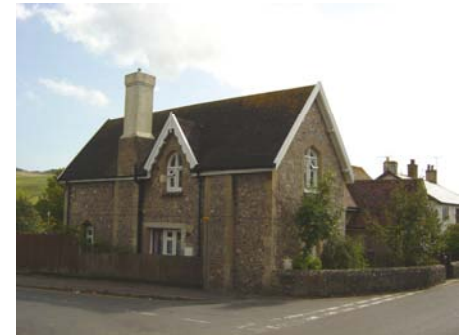
Fig 12. Former primary school
