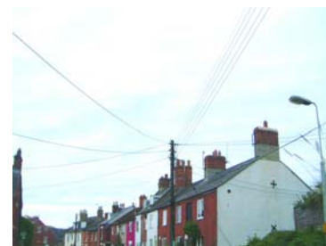
Fig. 59 Poles and wires detract from views, the street scene & the form of buildings
