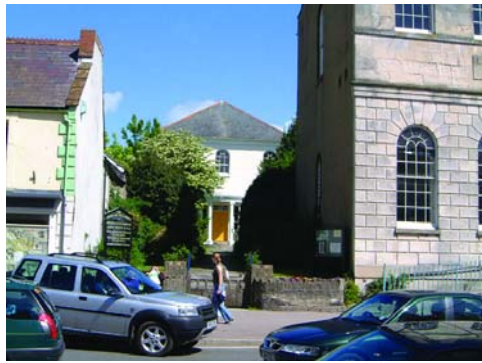
Fig. 15 The 'Chapel in the Garden' (Unitarian) set back from the general building line in East Street but still retaining its traditional boundary wall
