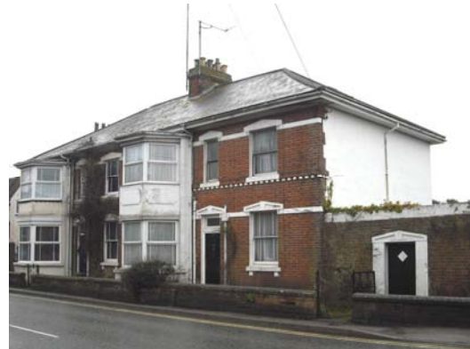
Fig D Nos 166 & 168 St Andrew's Rd
