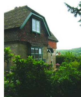
Fig.33 Right, former lodge to Downe Hall
