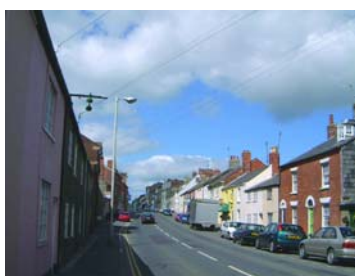
Fig. 57 Large lamp posts in East Street are visually intrusive
