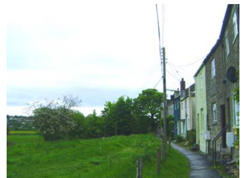
Fig. 27 South Mill Lane & its green foreground
