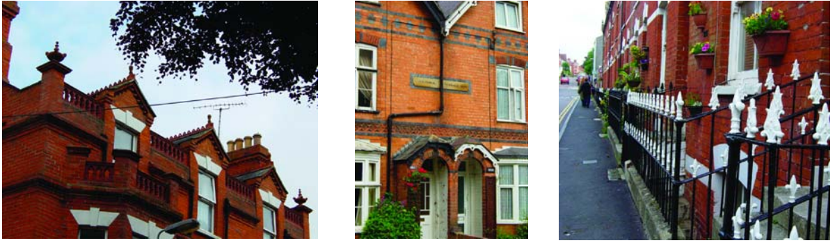
Fig. 37 Red/orange brick, slate, decorative timberwork and iron railings are typical of the materials and details in Victoria Grove
