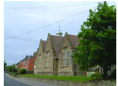
Fig. 29 The former school at the northern 'gateway' into St Andrew's Road
