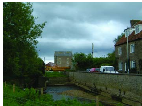
Fig. 25 View of South Mill from Asker Meadows
