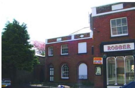
Fig. 50 The front of Nos. 27 & 29 West Allington
