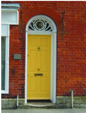
Fig. 6 Decorative fanlight, local brick & Bothenhampton stone plinth
