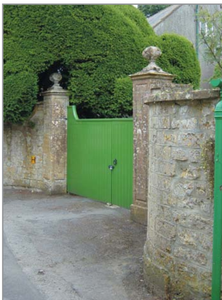
Fig.33 Wall and gate piers of Knowle Cottage
