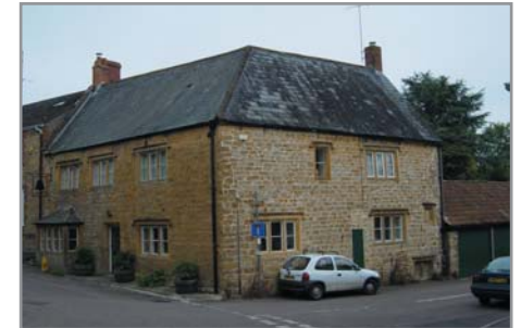
Fig.34 Former Eight Bells, 5 Church Street
