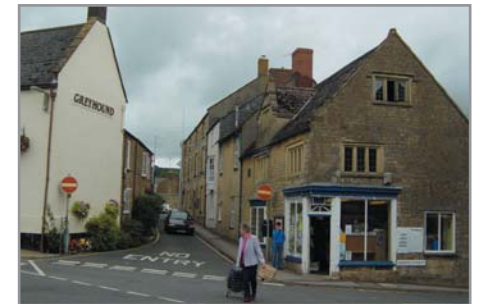
Fig.30 Corner shopfront of 12 The Square
