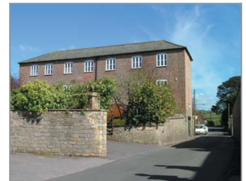
Fig.9 Former Mill, Whitcombe Lane
