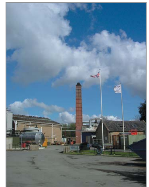
Fig.39 The Danisco Beaminster Ltd chimney is a landmark feature
