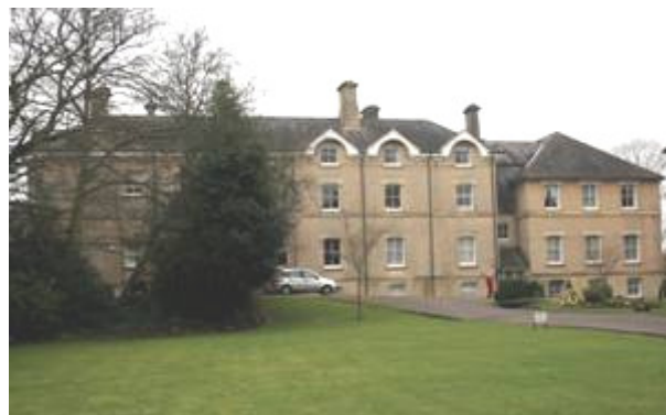
Figure 61: Westfield House, Redcott's Lane
