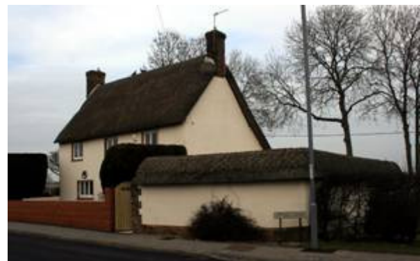
Figure 28: Angel Cottage , Stone Lane; 18 th century house with contemporary cob boundary wall
