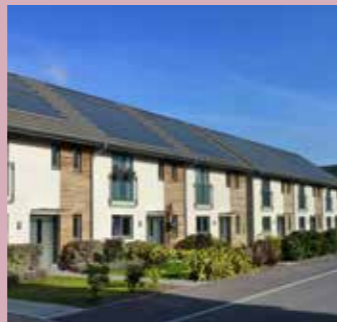
A strong building line defines the edge of the space
