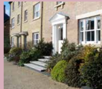
Windows and doors are placed to create an active frontage whilst maintaining some privacy through a set back
