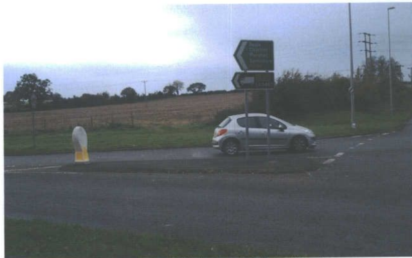
Figure 3-8: A350 Approach to Roundabout
