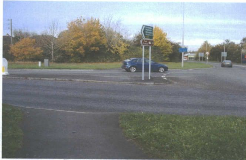
Figure 3-9: A354 Approach to Roundabout
