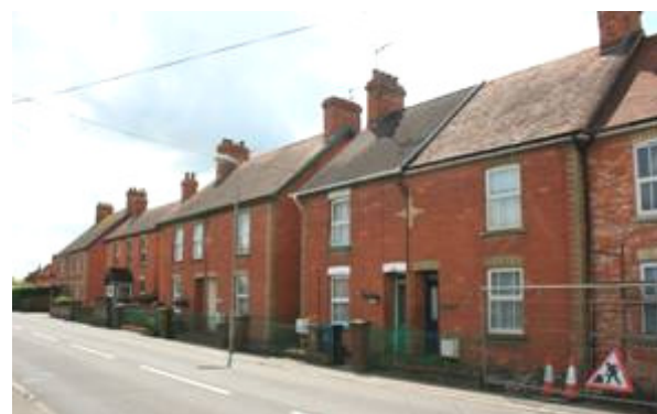
Figure 69: A row of 19 th century semi-detached houses on Shaftesbury Road, Ham.
