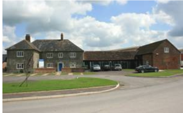
Figure 71: Park Farm, Kingsmead Business Park.
