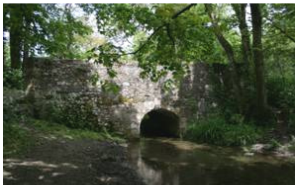
Figure 42: View of the 17 th century or earlier Kettle Bridge, Kettle Lane.
