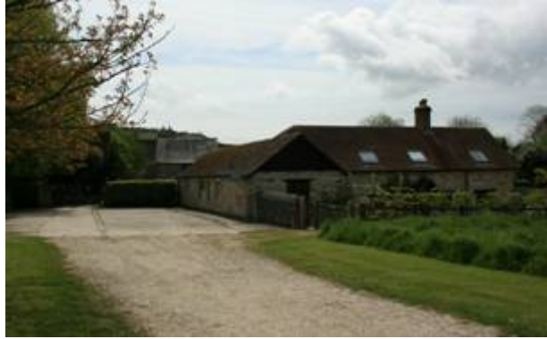
Figure 19: Abbey Farm outbuildings looking south.
