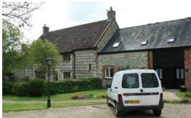
Figure 20: Mid-18th century Barton Farmhouse and attached barn.
