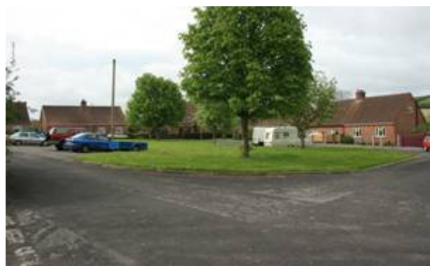
Figure 36: View of the post-war housing estate at Chescombe .
