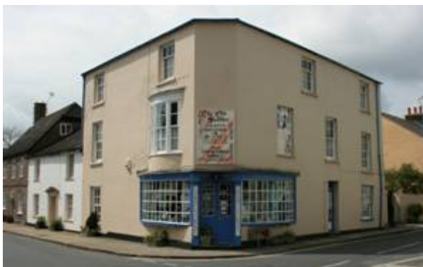
Figure 30: The Old Saddlery at the junction of Long St and Duck St, with its 19 th century shop frontage.
