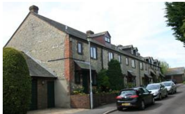
Figure 34: View of The Maltings, Acreman Street .
