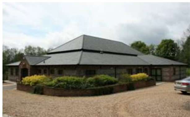
Figure 35: View of the new Village Hall, Kettle Lane.
