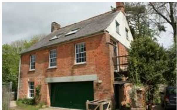
Figure 17: The 18 th century Mill House, Mill Lane.
