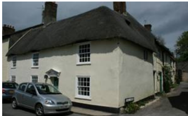
Figure 21: View of the 17 th century Old Forge and attached schoolhouse, with 18 th century re-fenestration.
