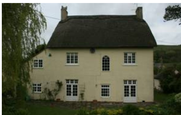
Figure 28: The south front of The Lodge, Alton Lane.
