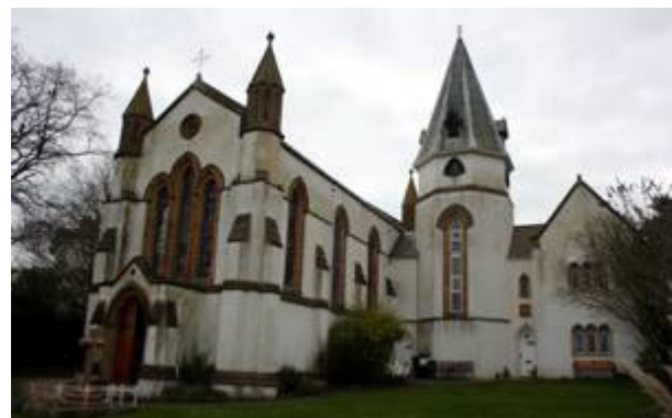
Figure 80: St Michael's and St George's RC Church, Silver Street.
