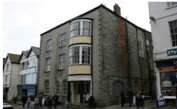
Figure 59: Former Three Cups Hotel, Broad Street.
