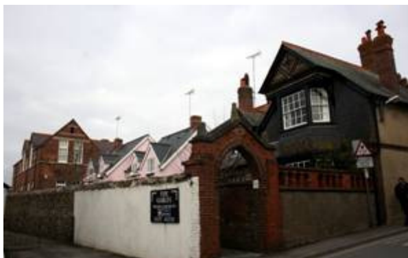
Figure 24: St Michael's School (left) and master's house, (right), Church Street.
