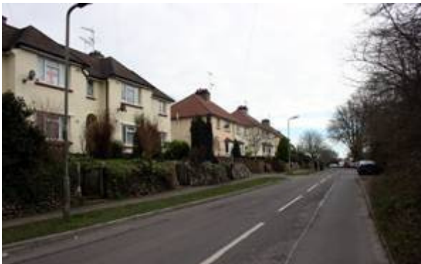
Figure 28: Council Houses, South Avenue, Colway Mead.
