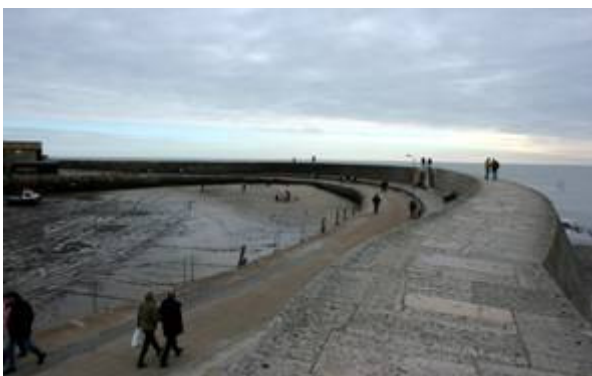
Figure 14: View along the Cobb, showing rebuild of 1824/5 in large Portland stone blocks.
