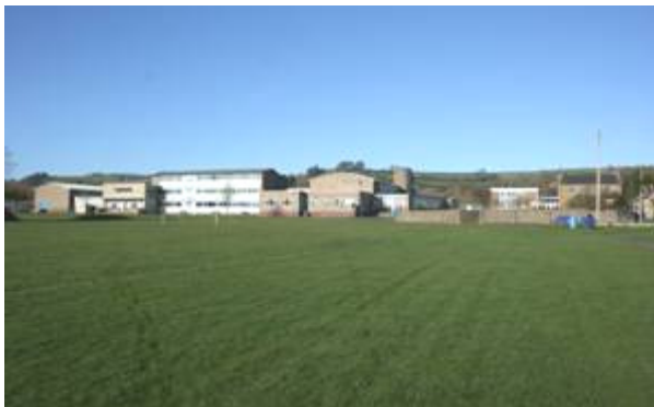
Figure 121: Beaminster School, viewed from south.
