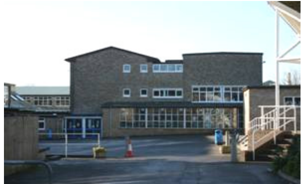
Figure 126: Beaminster School buildings, viewed from east.
