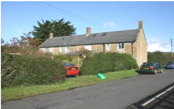
Figure 85: 19th century terraced cottages on Bowgrove Road.
