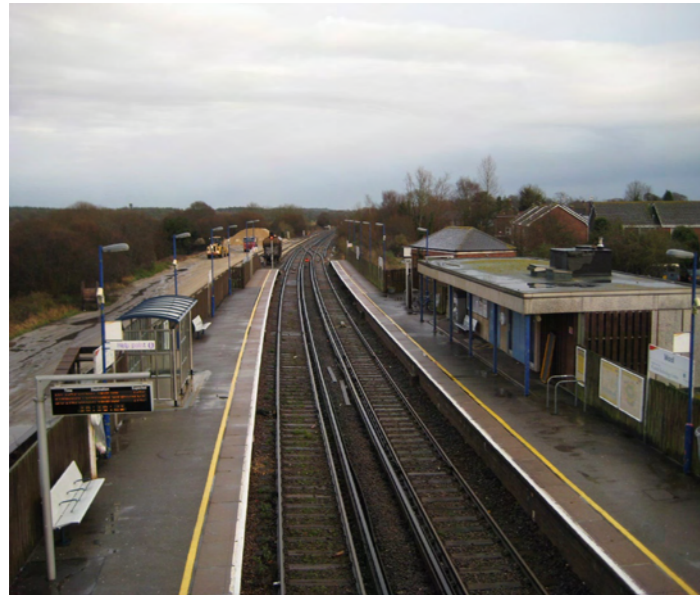
1. The railway station is an important asset to the village and provides an alternative means of transport to the private car.
