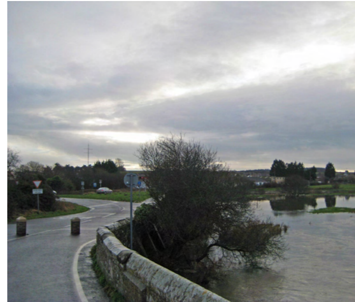
1. View south towards Wool from the original historic bridge over the River Frome.
