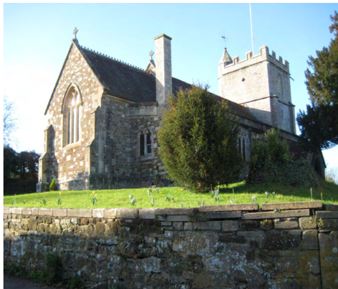
3. The church is one of a number of listed buildings owing its architectural and historic interest.
