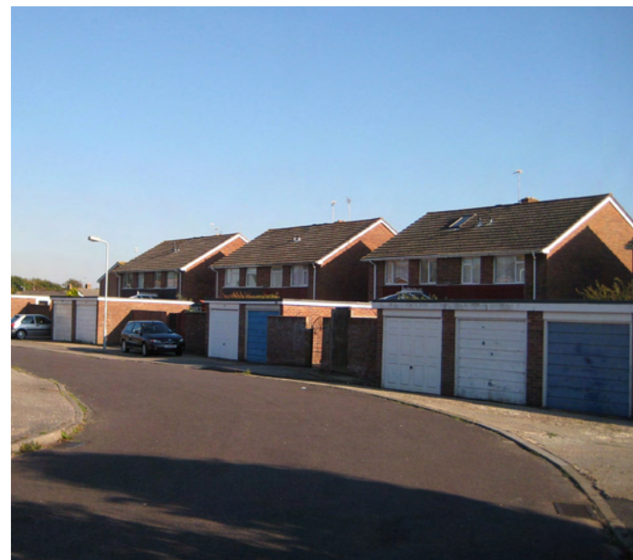
3. Many residential areas have garaging and parking directly addressing the street. This is unsightly and forms negative areas of townscape.
