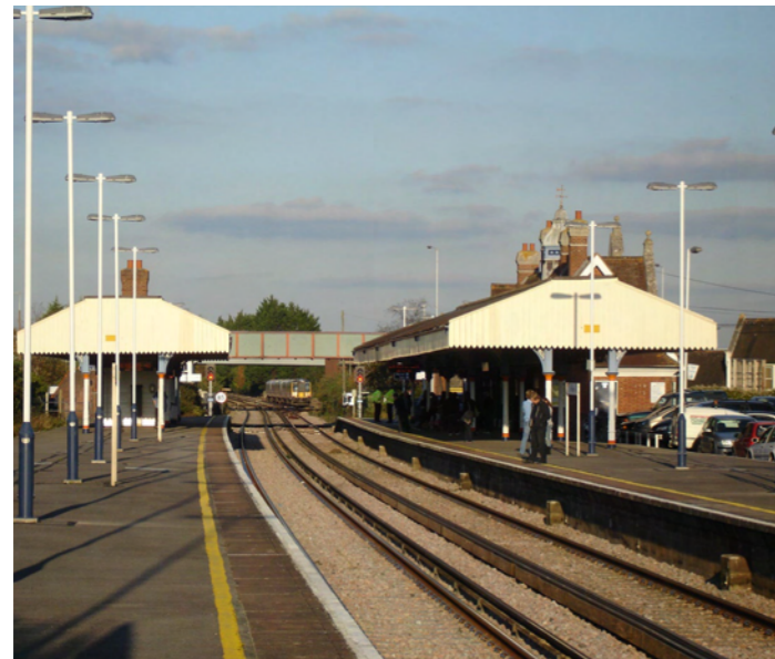
1. The railway station generates activity and provides something of a focal point for the settlement.
