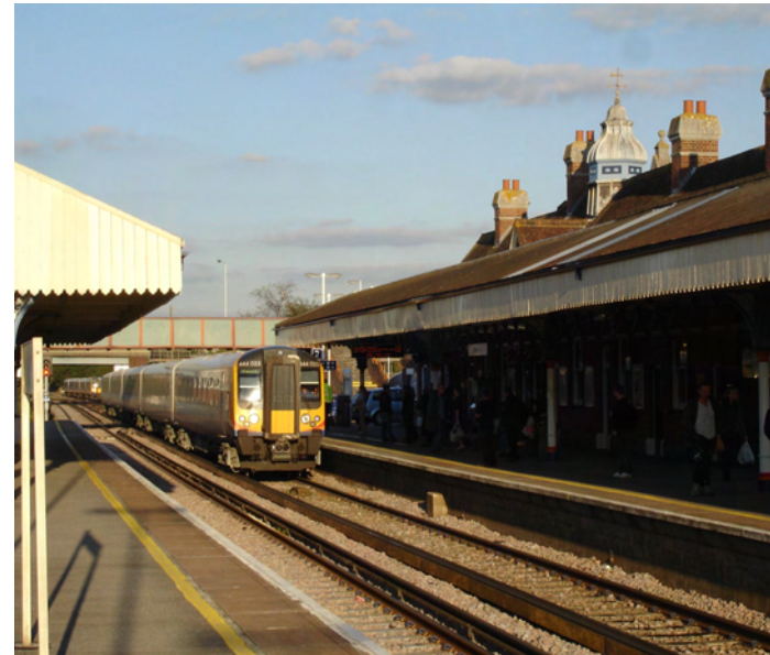
1. The railway is one of the settlement's most important uses and generates both interest and vitality.
