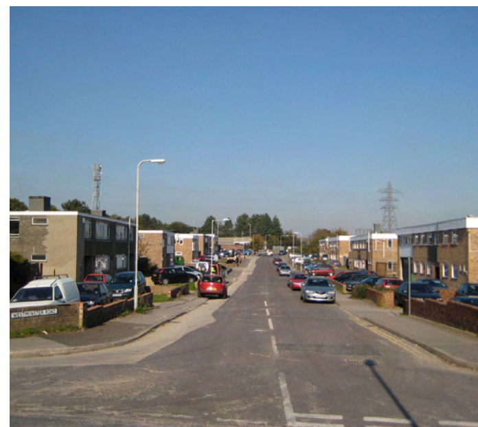
4. Three industrial estates provide important employment land, but are unsightly areas of townscape.
