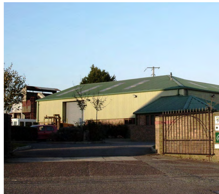
3. The largest scale buildings are located on the industrial estates at the edges of the settlement.
