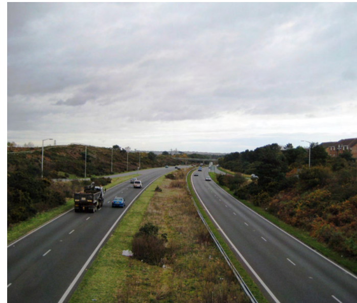
2. The A35 dual carriageway forms a clear edge to the town and is the main road connection for Upton.
