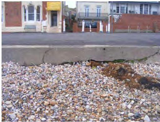
Figure 3-14 Concrete wall constructed as part of previous widening of the promenade between Greenhill Gardens and Pier Bandstand (23-11-2018; photos by A. Frampton).
