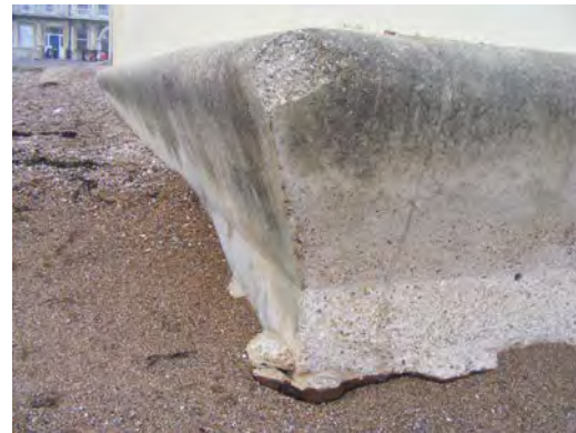
Figure 3-13 Tops of sheet piles exposed at southern end of the Pier Bandstand (23-11-2018; photos by A. Frampton).
