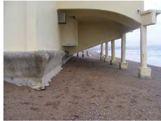
Figure 3-12 Photos of the Pier Bandstand seawall and how it protrudes into the intertidal area of the beach (see bottom left photo in particular) (23-11-2018; photos by A. Frampton).
