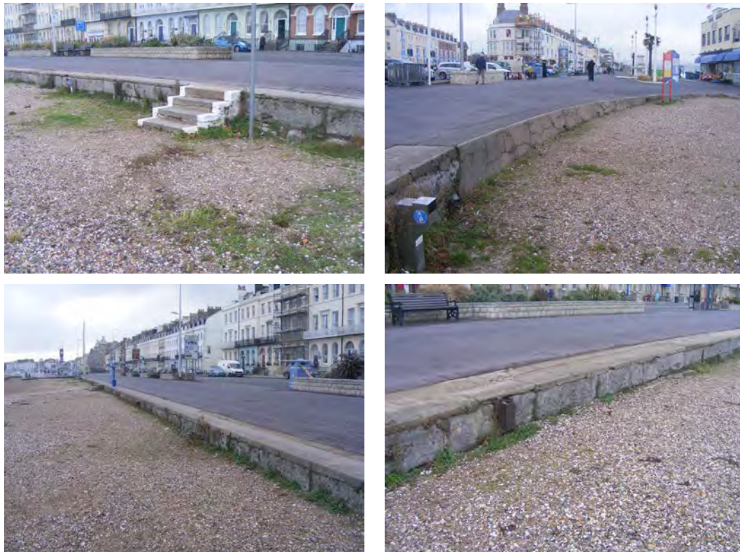
Figure 3-11 Photos of the promenade and masonry block wall between Jubilee Clock and Pier Bandstand, showing concrete topping original masonry blocks (23-11-2018; photos by A. Frampton).
