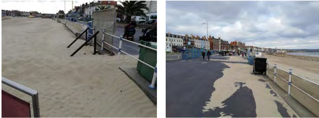
Figure 3-5 Evidence of wind-blown sand pushed up against the promenade/seawall, covering access step; also shown is sand netting placed along railings in this area each autumn/winter to reduce amount of sand blowing further landwards and evidence of wind-blown sand on the promenade (14-12-2018; photos by A. Frampton).
