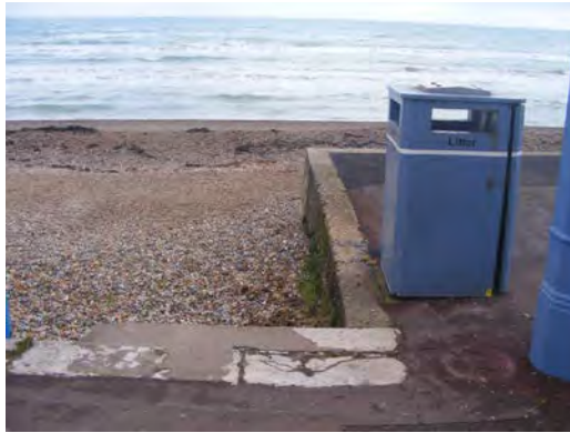
Figure 3-14 Concrete wall constructed as part of previous widening of the promenade between Greenhill Gardens and Pier Bandstand (23-11-2018; photos by A. Frampton).
