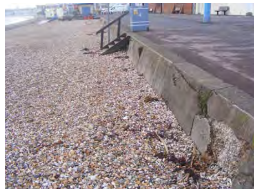
Figure 3-15 Poor condition of concrete including evidence of voids along parts of the concrete wall between Greenhill Gardens and Pier Bandstand (23-11-2018; photos by A. Frampton).
