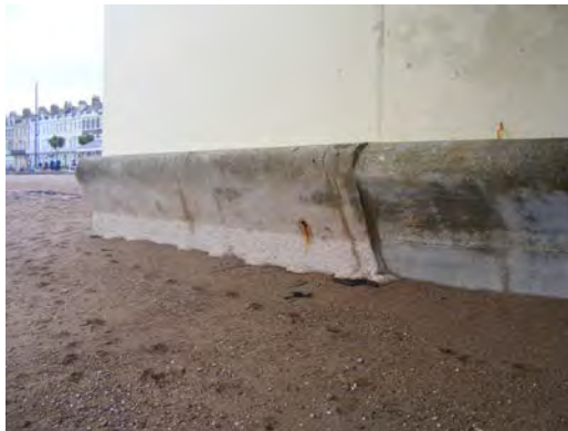
Figure 3-13 Tops of sheet piles exposed at southern end of the Pier Bandstand (23-11-2018; photos by A. Frampton).
