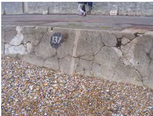
Figure 3-15 Poor condition of concrete including evidence of voids along parts of the concrete wall between Greenhill Gardens and Pier Bandstand (23-11-2018; photos by A. Frampton).
