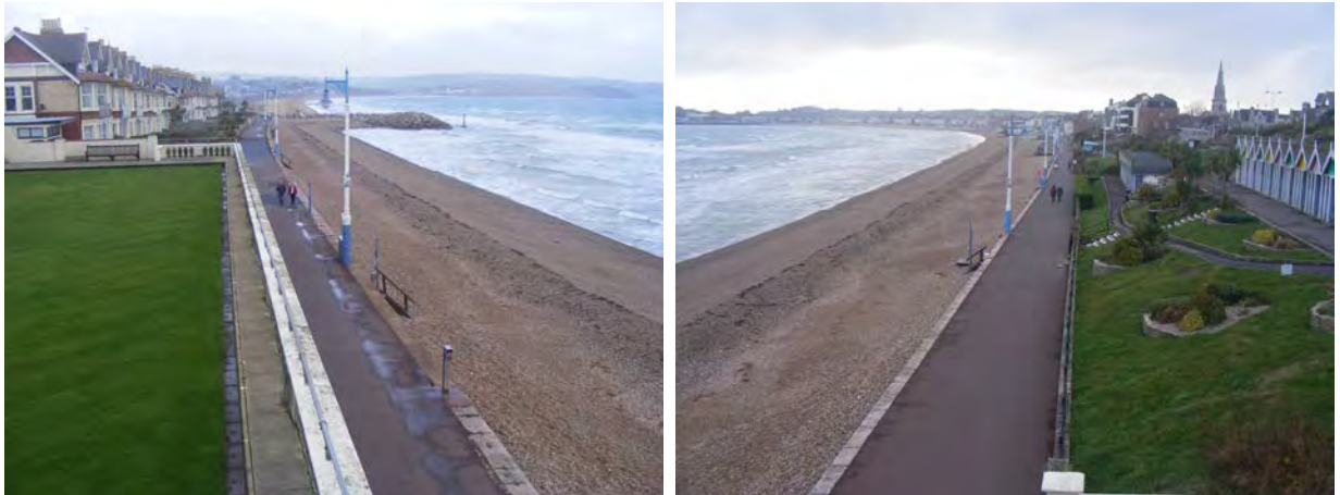
Figure 2-6 Views along the Greenhill Beach section of frontage to north (left) and south (right) showing the narrower and steeper shingle upper beach (compared to beach shown in Figure 6-2) leading to flatter and sandier foreshore (23-11-2018; photos by A. Frampton).
