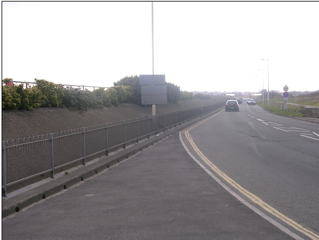
Photo 4.2 Preston Beach Sea wall
