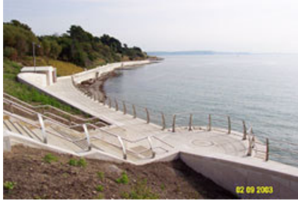
Photo 4.3 Newton's Cove coastal protection scheme
