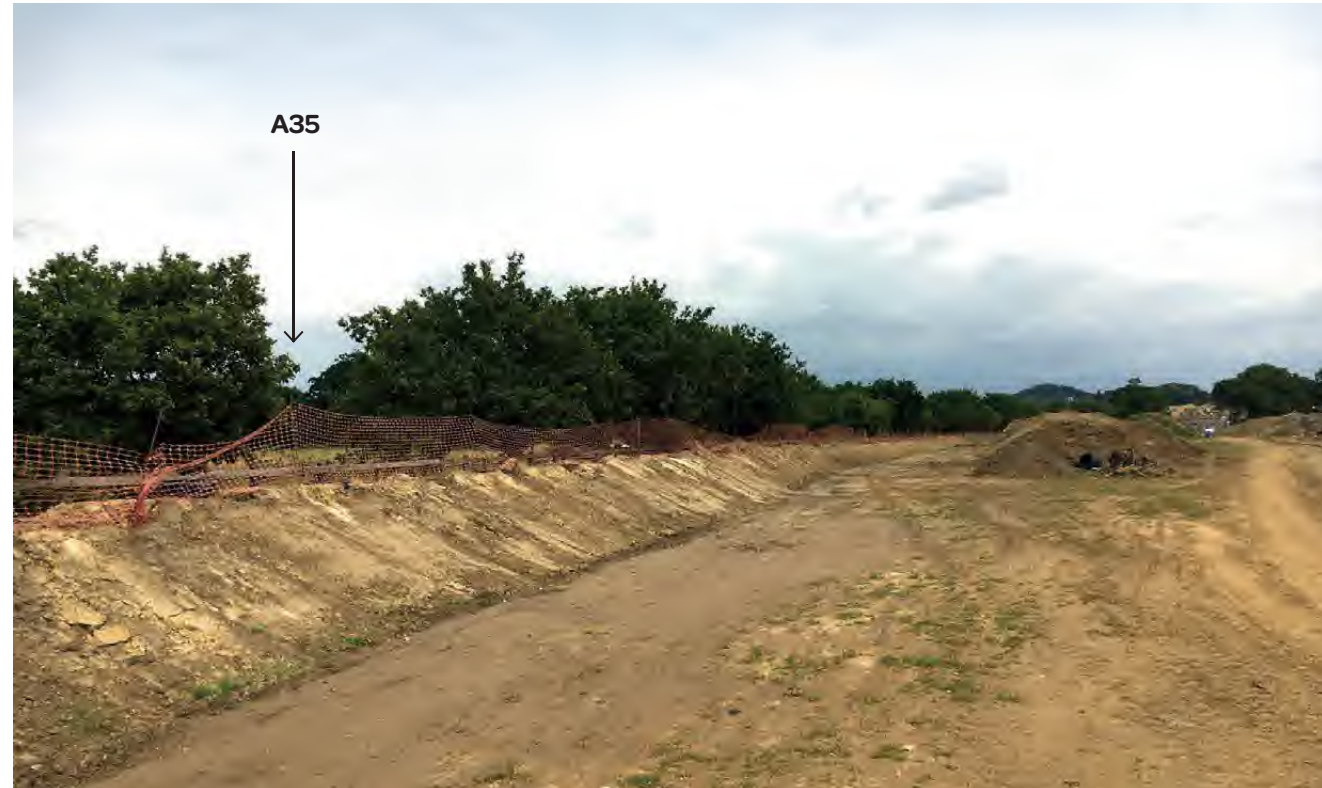
View looking north over noise bund under construction
