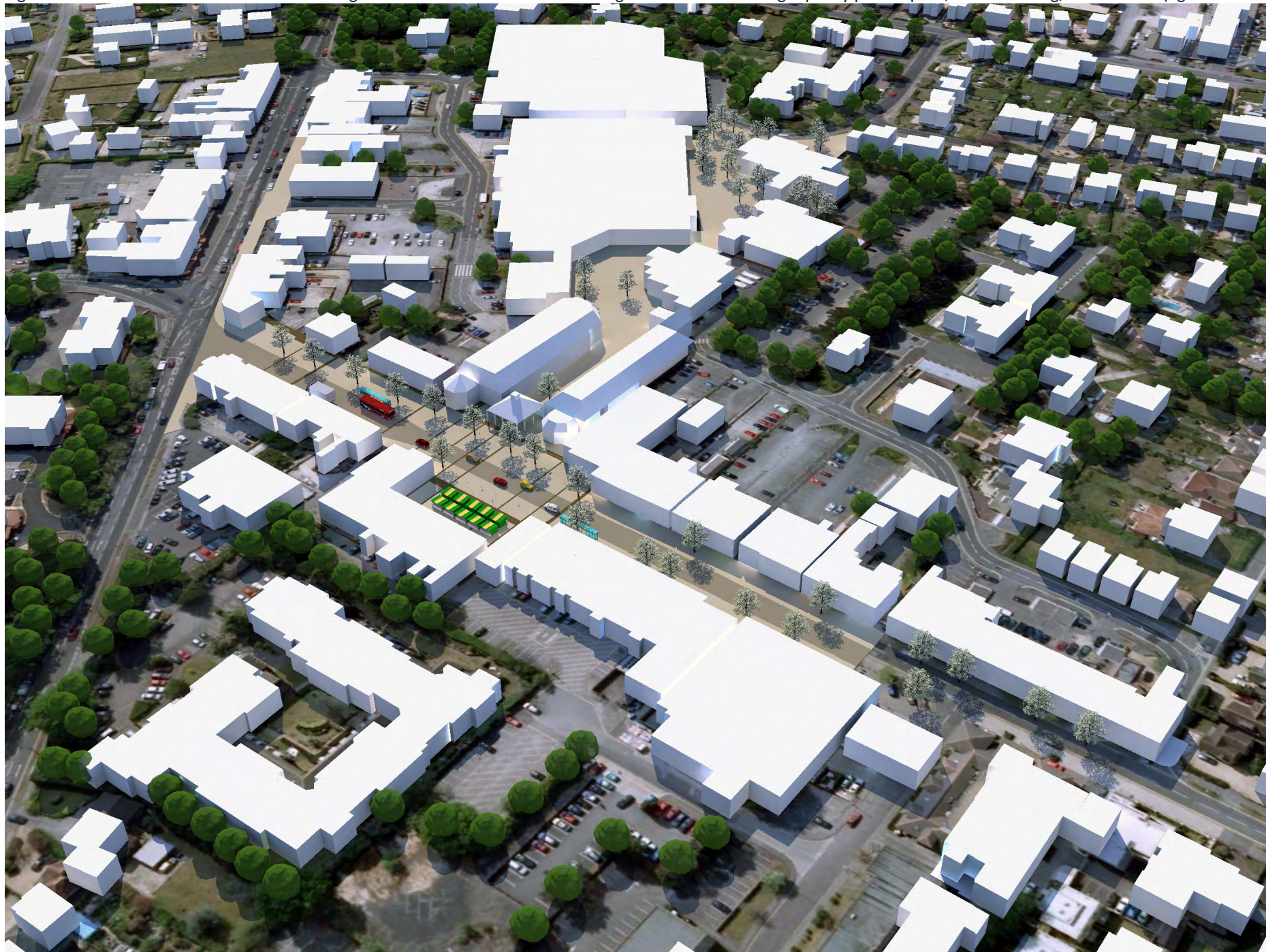
Figure F3: Ferndown - create a more welcoming entrance to the town centre through the creation of a high quality public space, traffic calming, flexible uses (eg farmers market/parking)
