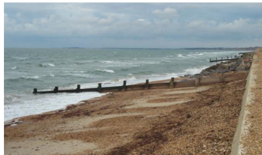
Figure 1.2 Timber groyne & seawall at Milford-on-Sea
